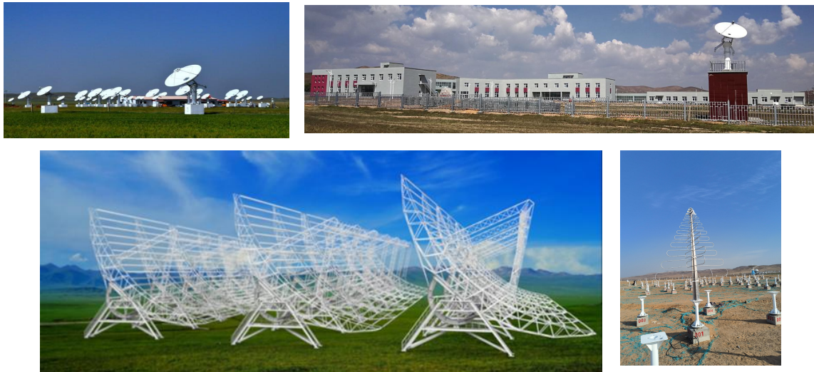
Figure 1. Up left panel: Central part of MUSER arrays; Up right panel: Mingantu Observing Base buildings; Lower left panel: Design of three 140m×40m cylinder antennas; Lower right panel: Construction process of extension of MUSER in decametric waverange.
