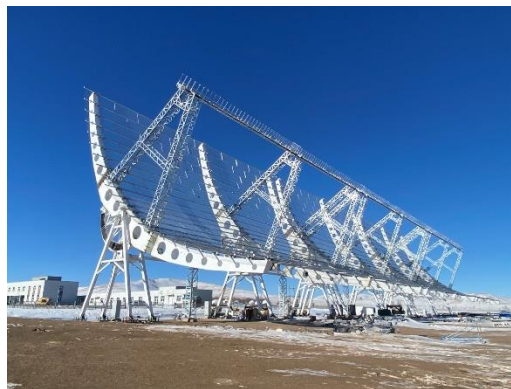
Figure 1. The parabolic cylinder antenna of IPS telescope
