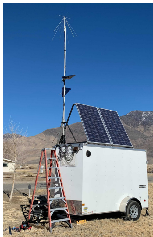
(a) Outside view of the RFI monitoring station.
