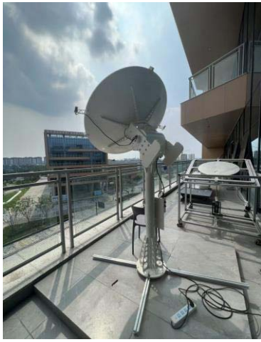
Figure 3. Align the antenna with the sun for overall system testing
