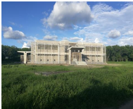
Figure 8. Front side view of Multi purpose building (MPB) shielded structure .
