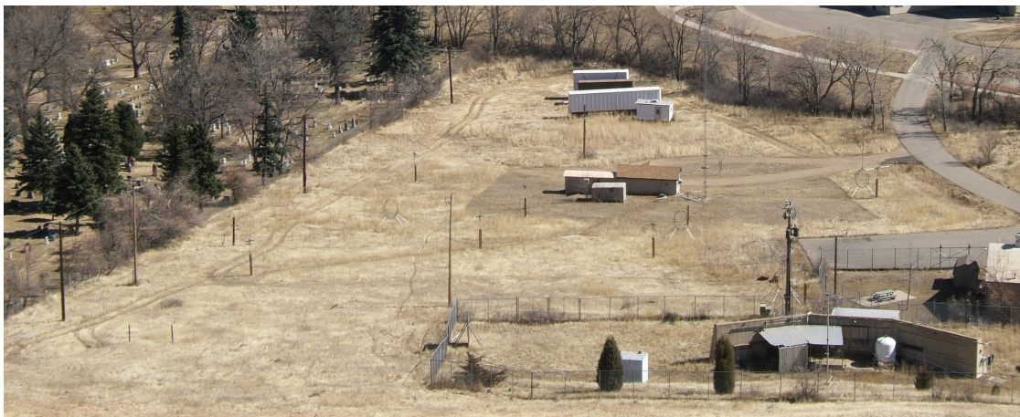
Figure 2: Boulder Ionosonde Station, March 2006
