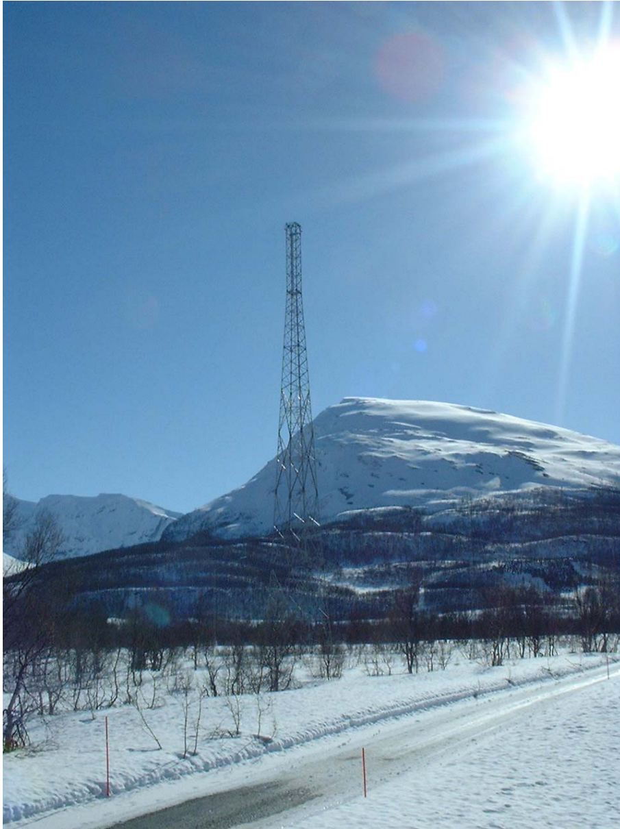
Fig. 8. The current transmitter antenna arrangement at Ramfjordmoen. (Photo: Chris Hall)
