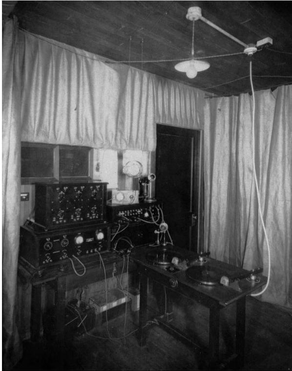
Figure 1. CKUA control room in 1932. Reproduced from [3].
