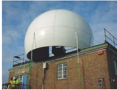
Fig. 2. The Raytheon control tower with the radome on the roof.
