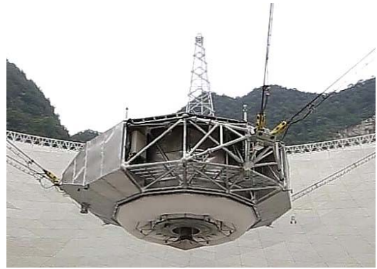
Figure 4. The photo of the feed cabin of FAST.
