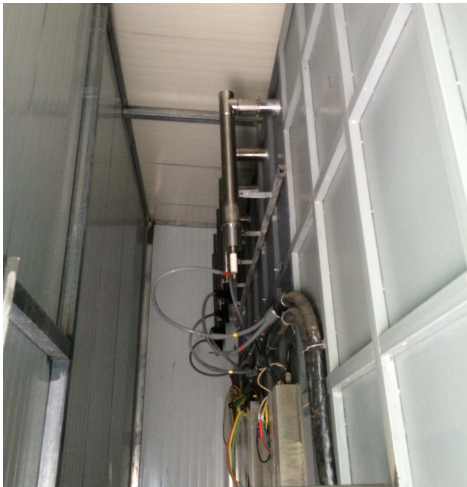
Figure 6. The photo of the 10 KV power filter installed at the shielded transformer substation.
