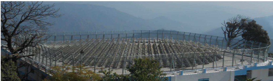
Figure 1. Antenna array on the roof-top of the ASTRAD building with clutter fence along the periphery of the antenna array.
