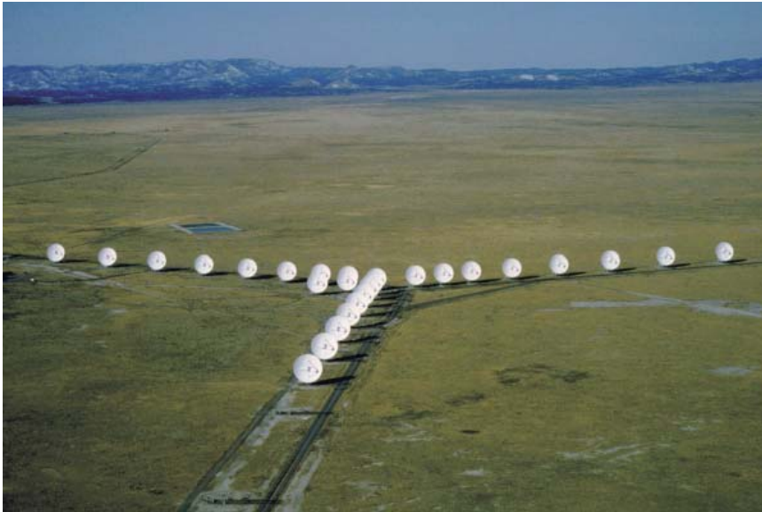
Figure 1. The Karl G. Jansky Very Large Array (VLA), located in central New Mexico, includes twenty-seven 25 m antennas, operating from a few hundred MHz to 50 GHz. Each antenna moves on railroad tracts along three arms to cover configurations ranging from 1 km to 36 km. The angular resolution at the shortest wavelength and in the largest configuration is 0.04 arcsec, about that of the Hubble Space Telescope.
