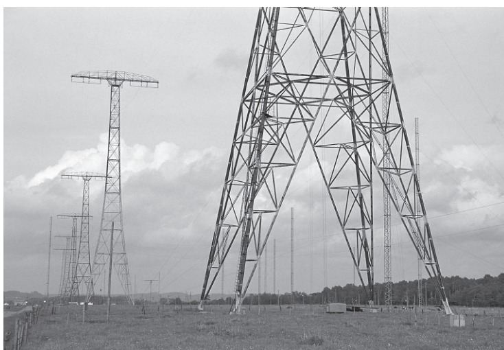
Figure 1. Some of the six 127-m-tall steel towers that support the transmitting antennas (photo by Bengt A. Lundberg, Swedish National Heritage Board).
