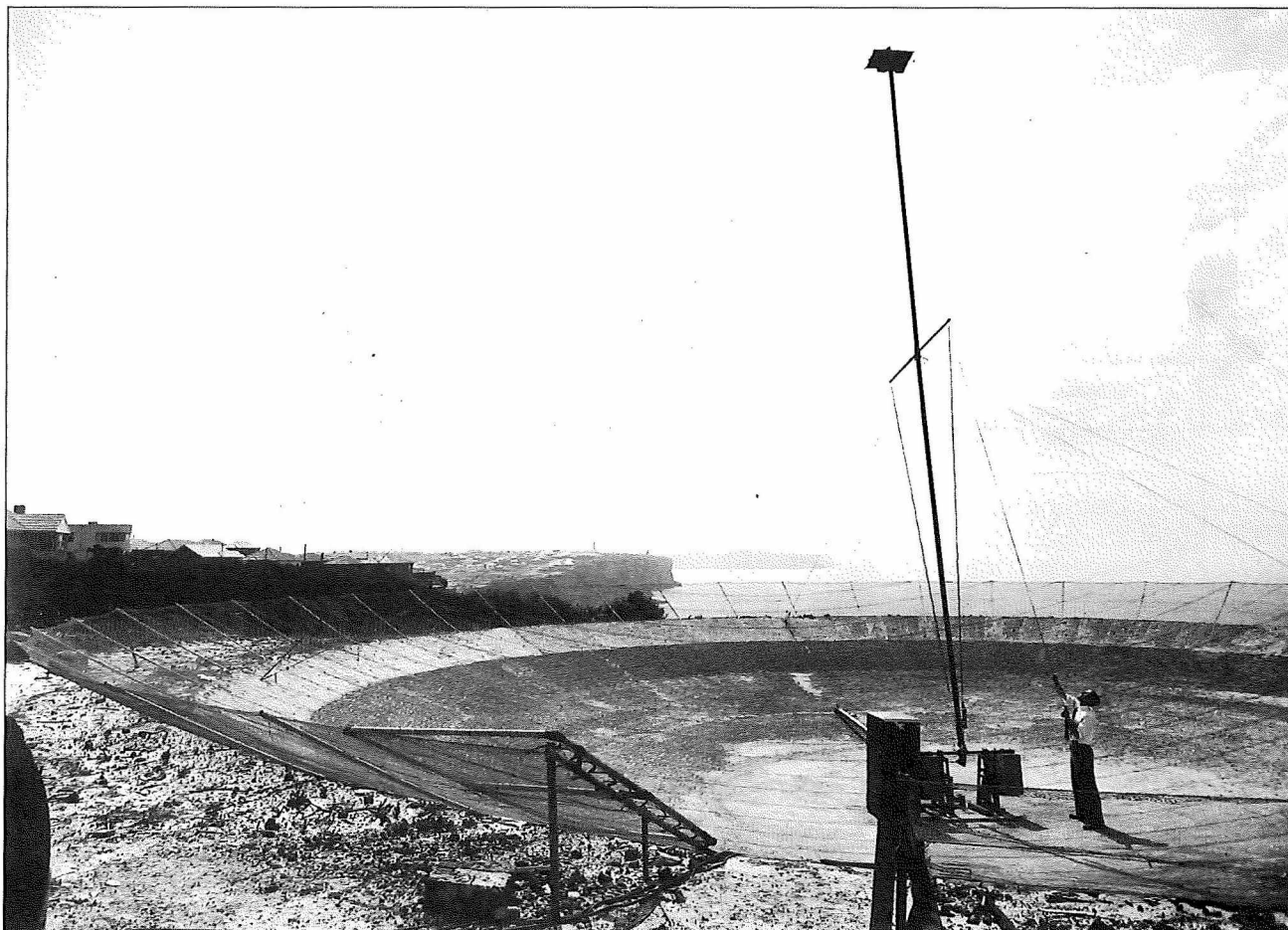
Figure 11. The complete 80-ft reflector showing the addition of the wire mesh surface, the feed mast and the housing for the second stages of the receiver at the vortex.
