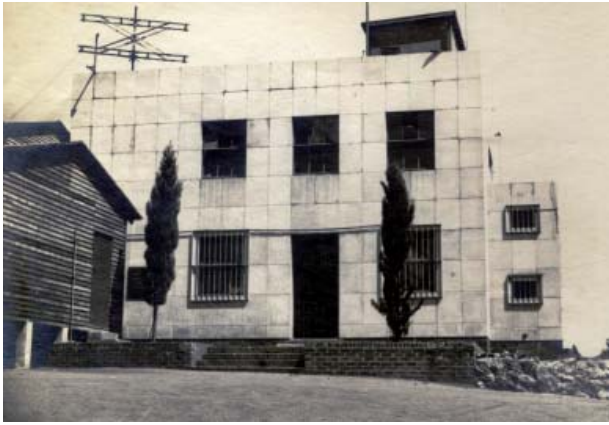
Figure 7. The BPI building, with a radar antenna on the roof.
